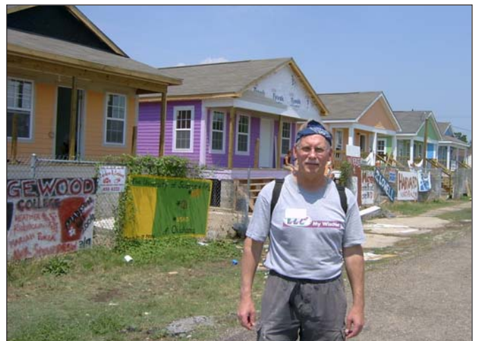
Bob Bocher stands in front of houses under construction in New Orleans' Upper Ninth Ward.
